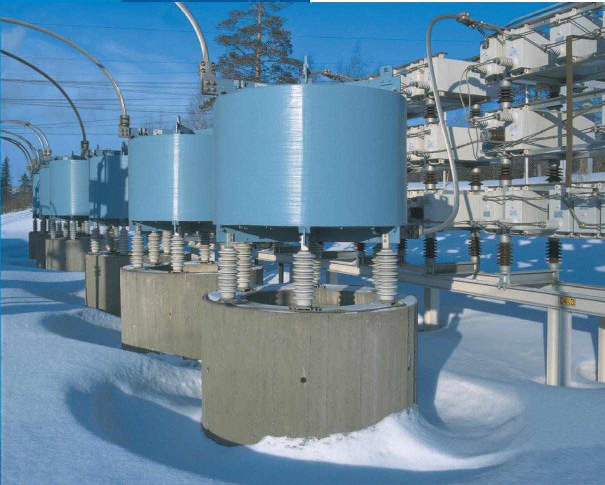
However, when non-linear loads - such as thyristor drives, converters and arc furnaces - are connected to the system, excessive harmonic currents are generated, and this causes both current and voltage distortion. Harmonic filtering is the best way to eliminate this distortion from the power system.
